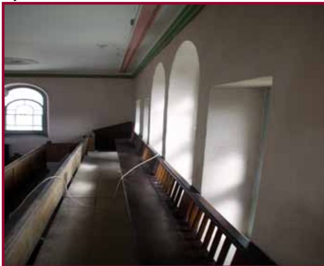
Hen Dŷ Cwrdd: repairs to historic fabric
